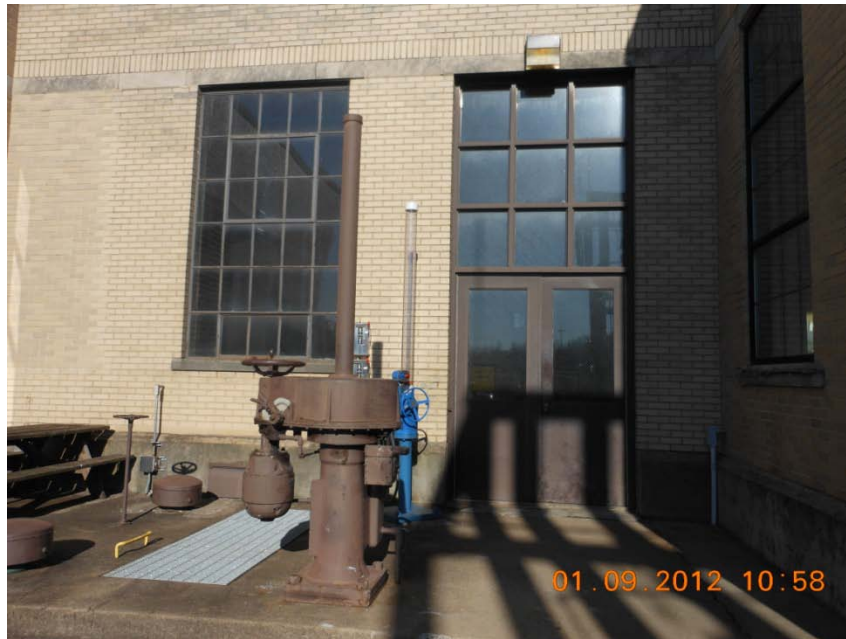
South Elevation, Door Area
